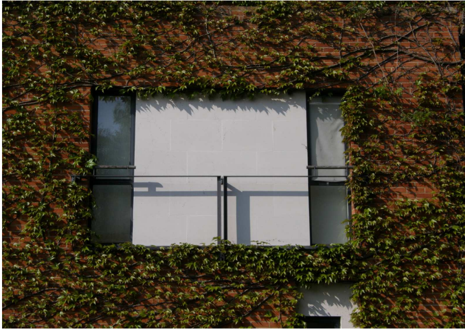
Fig. 33 — The South Wall of the Rosalind Franklin Building
