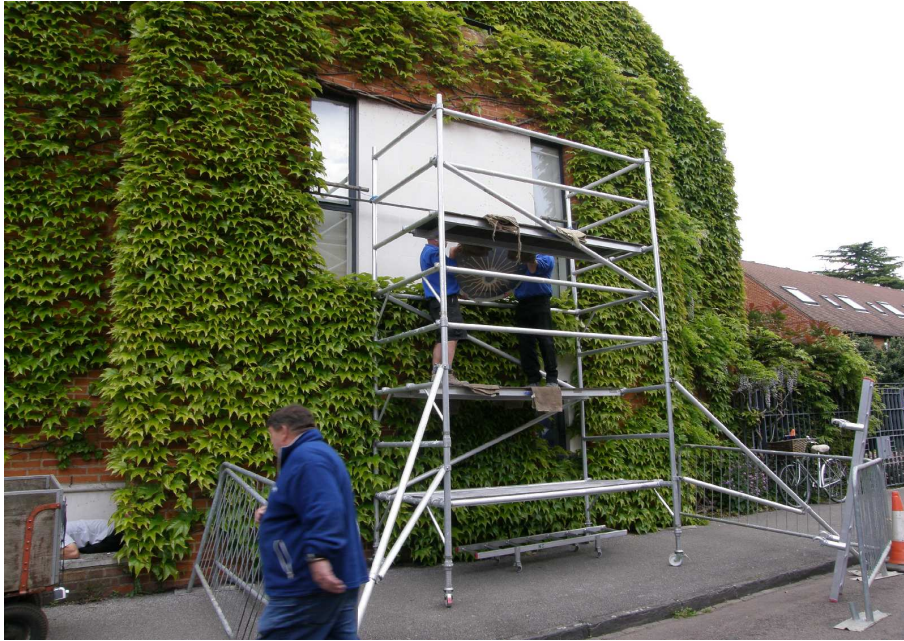
Fig. 54 — Kevin and Michael lifting the Slate up the Scaffolding
